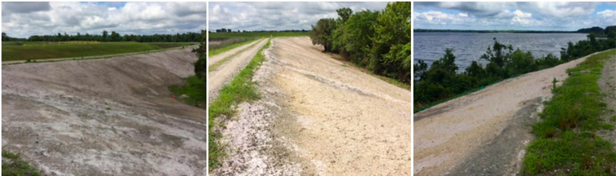
Coal Ash Containment: 3:1 Slopes covered with Posi-Lock™ after 1 year and 90" of rain!
